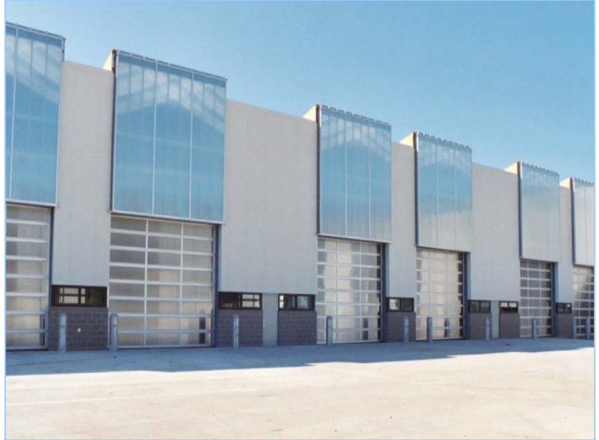
ID # 19001- CPI Daylighting provided over 27,000 sq. ft. of daylighting products for this Pennsylvania Army National Guard Unit Training Equipment Site.
